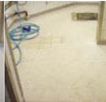
Pose carrelage et joints
